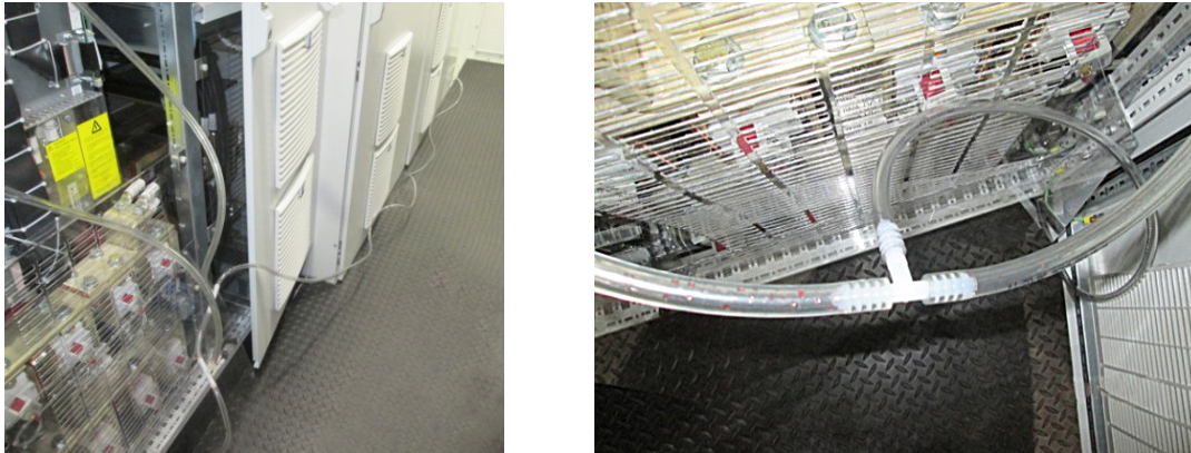
Figure 8: Connect bleed hoses together
