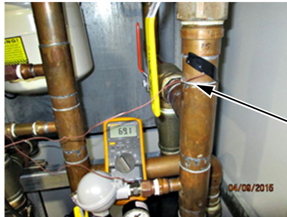
Figure 2: Thermocouple placement
